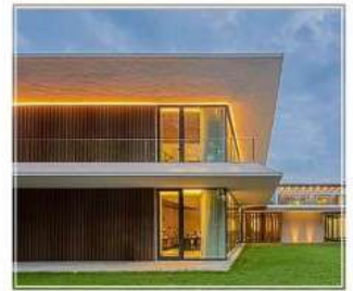
A facade design by ILDL, New Delhi. The lighting follows the building's architecture.
